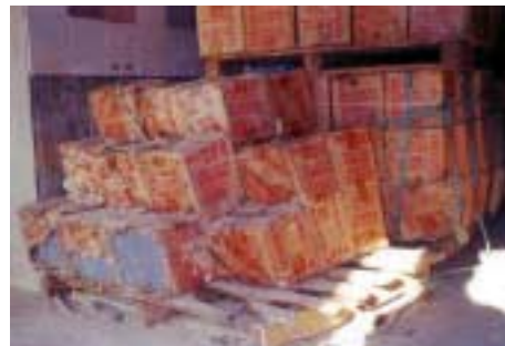
Figure 3.4 Improper stacking of tiles
