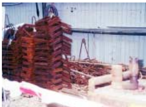
Figure 3.7 Cutting waste of reinforcement
