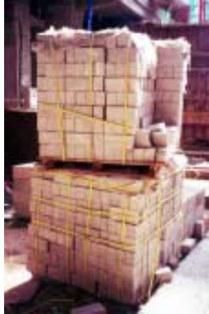
Figure 3.16 Stacking of blocks on pallet
