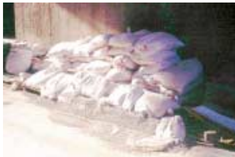
Figure 3.3 Broken bag of crush stone
