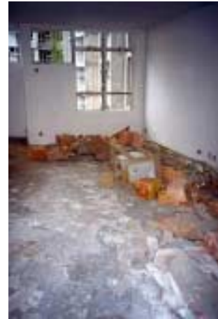
Figure 3.14 Cutting waste of tiles
