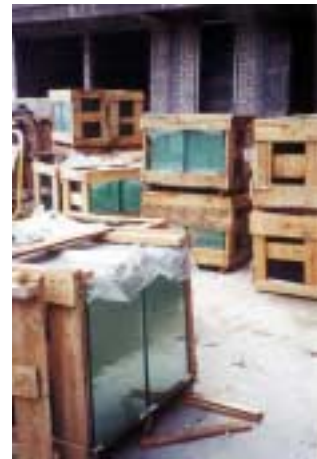
Figure 3.20 Storage of glass in wooden box
