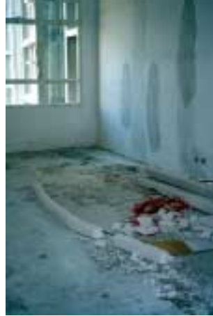
Figure 3.10 Cutting waste of dry wall
