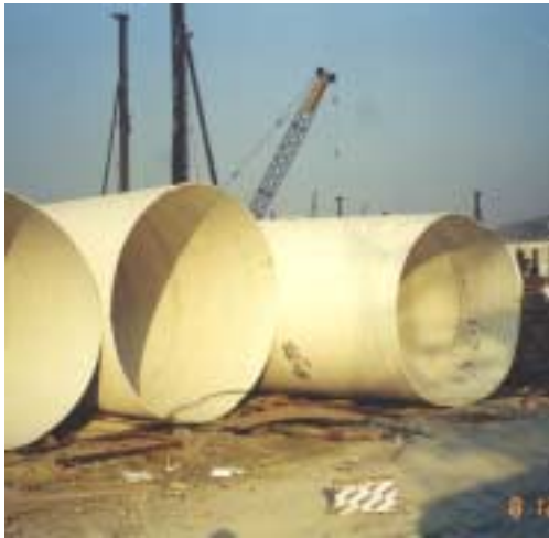
Figure 4.14 UPVC column forms
