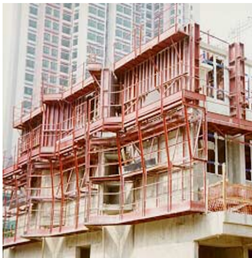
Figure 4.11 Large panel formwork
