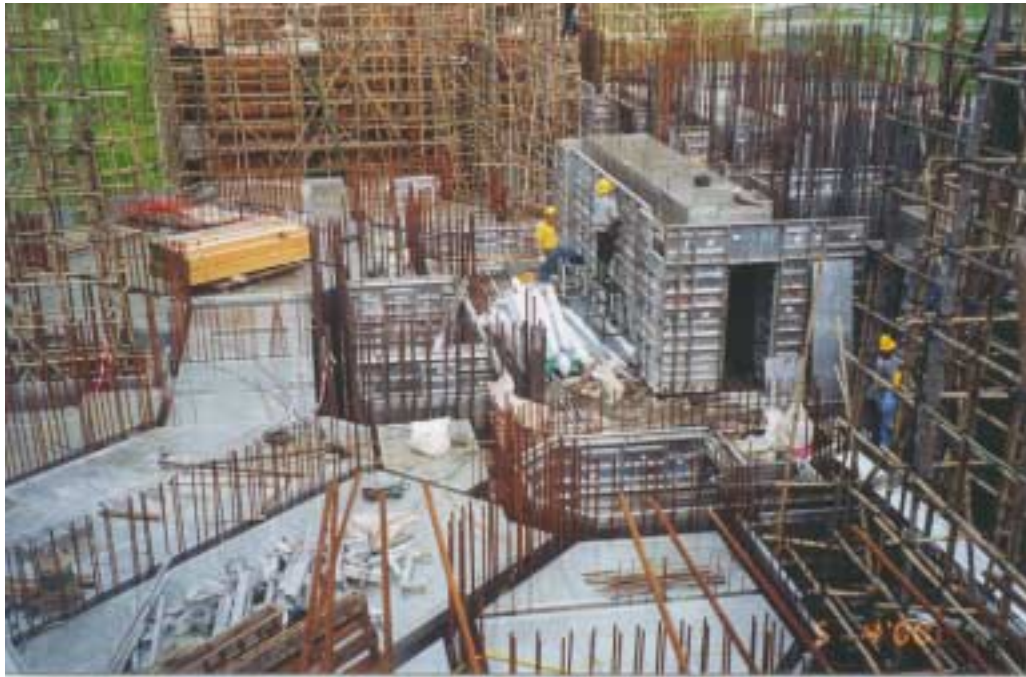
Figure 4.13 Installation of aluminum formwork
