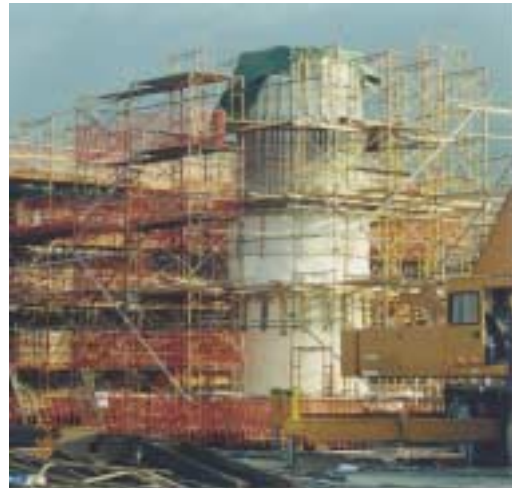
Figure 4.15 Erection of column forms
