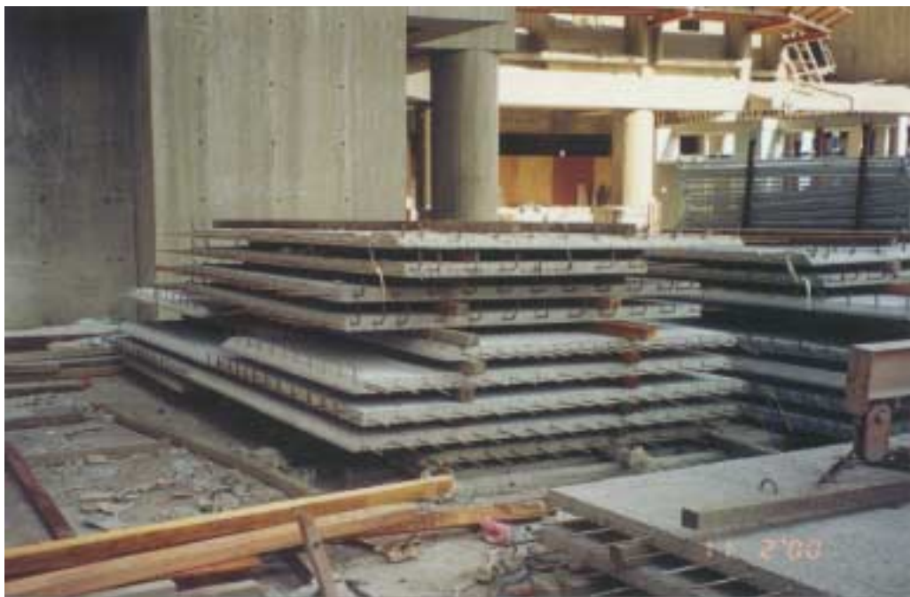
Figure 4.9 The lower layer of semi-precast slab
