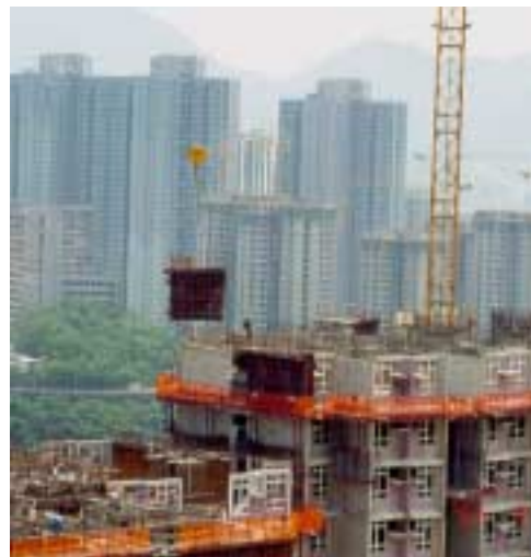
Figure 4.12 Removal of formwork
