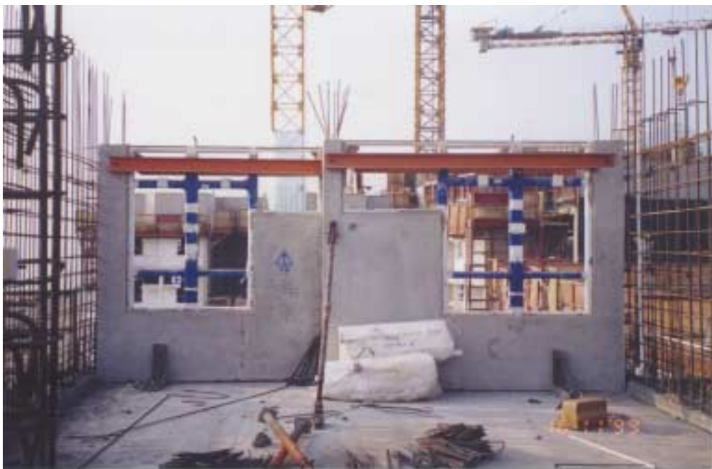
Figure 4.8 The precast façade is secured with temporary bracing
