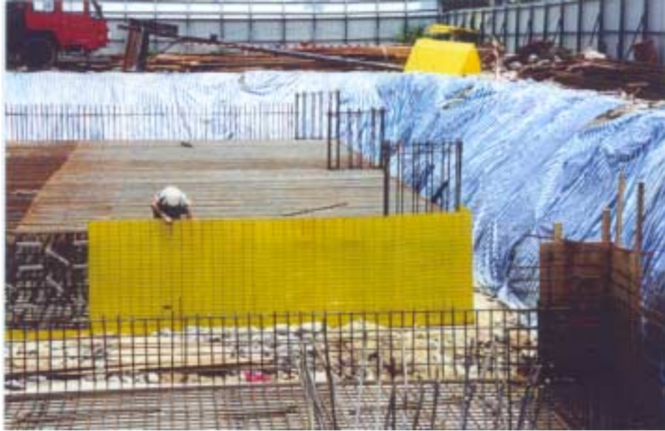
Figure 4.16 Construction of pile caps using Pecaform
