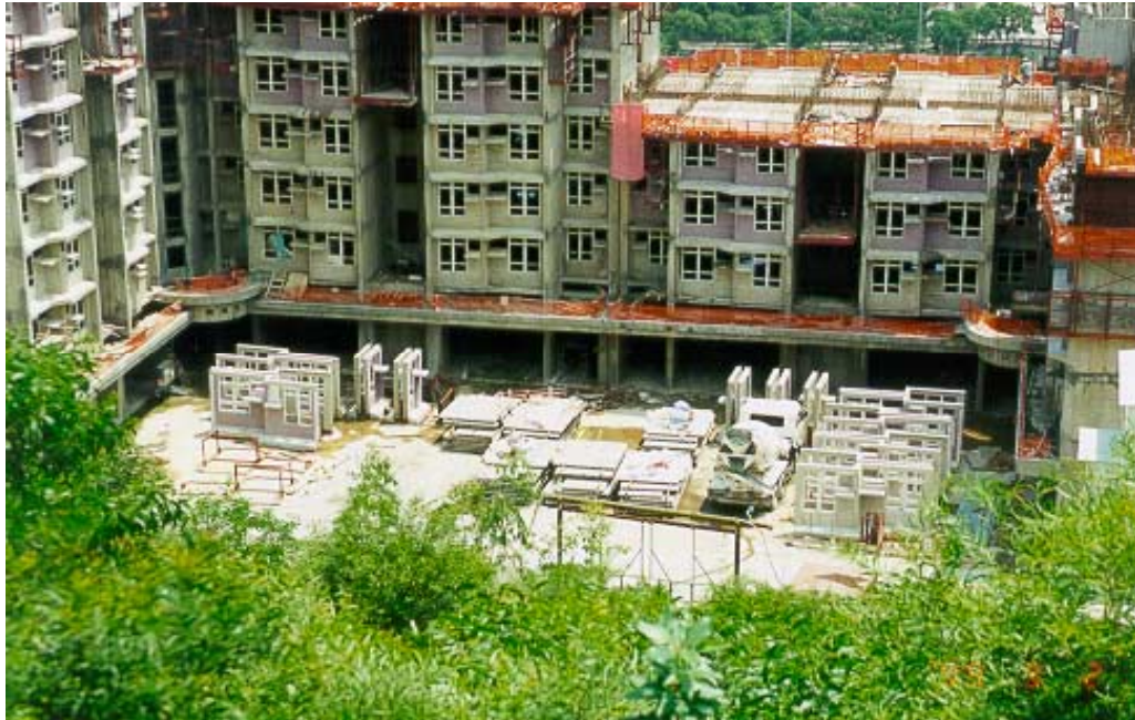
Figure 4.6 Prefabrication yard on site
