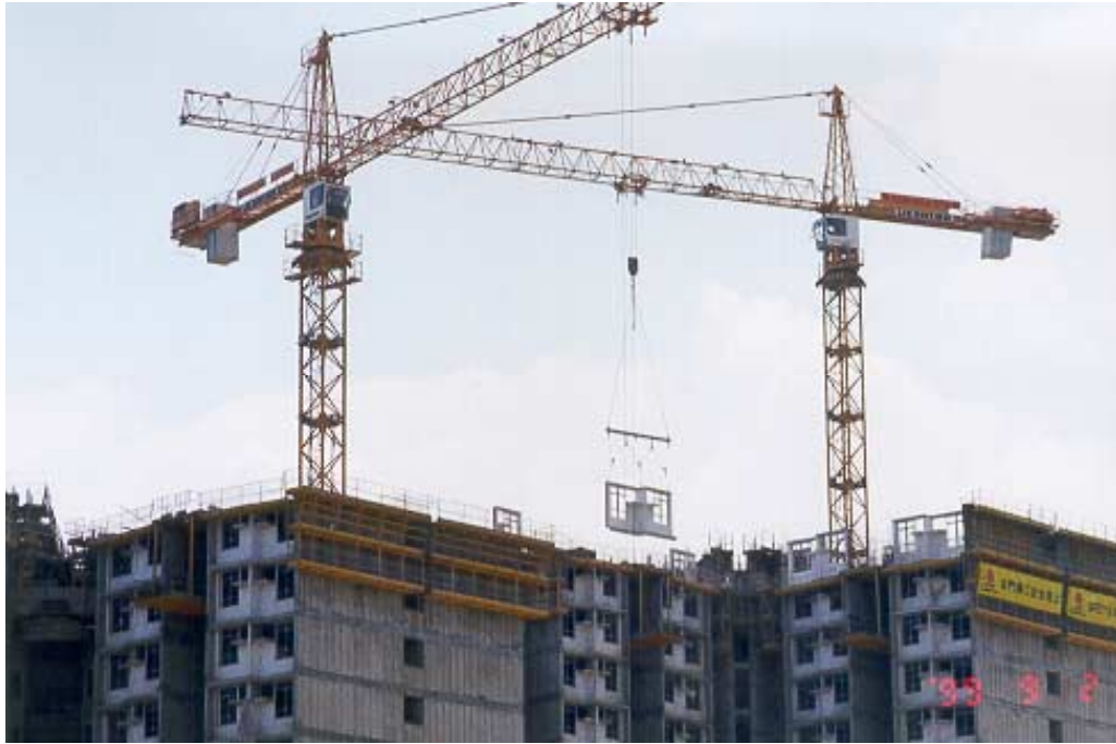
Figure 4.7 Transfer of prefabricated façade to the working level
