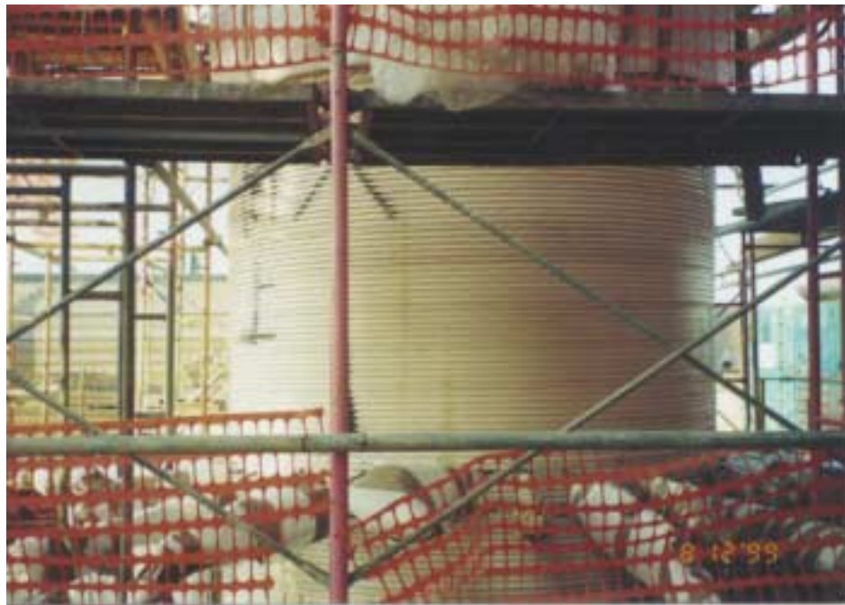
Figure 4.35 UPVC column formwork
