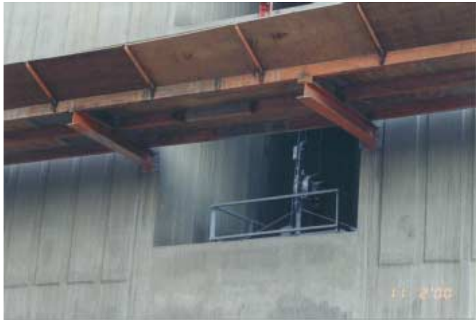
Figure 4.32 Gondola used for applying external finishes
