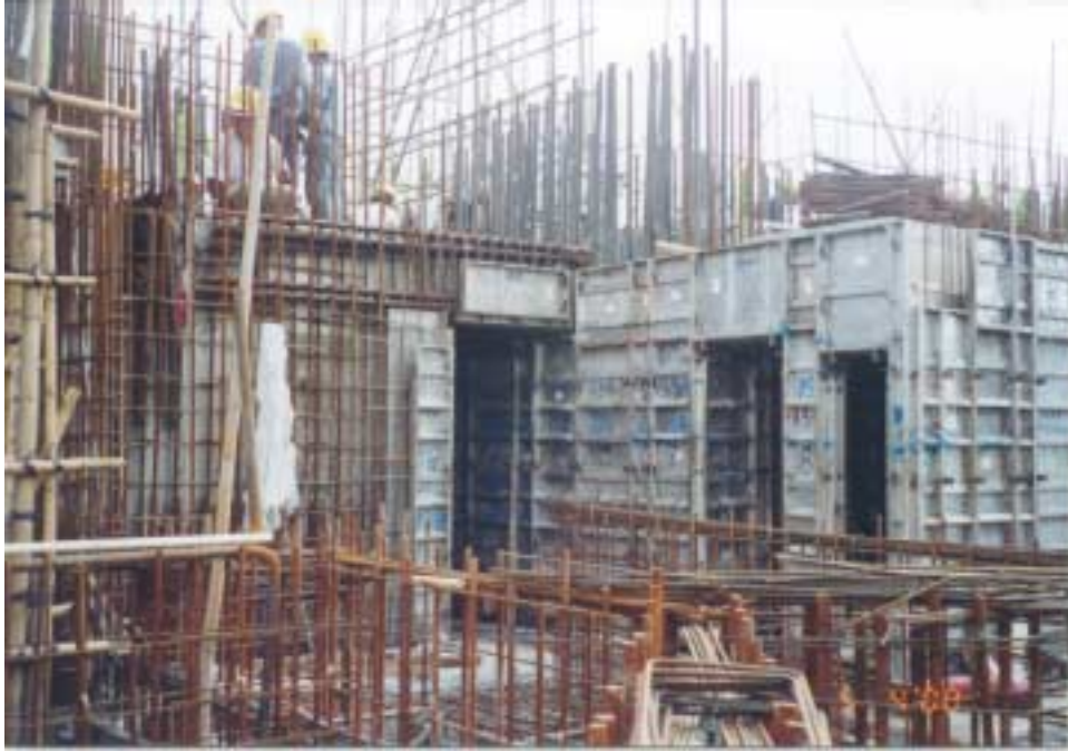
Figure 4.36 Aluminum Formwork
