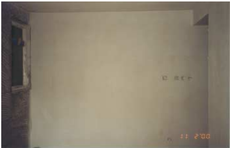
Figure 4.31 A wall finished by spray plastering
