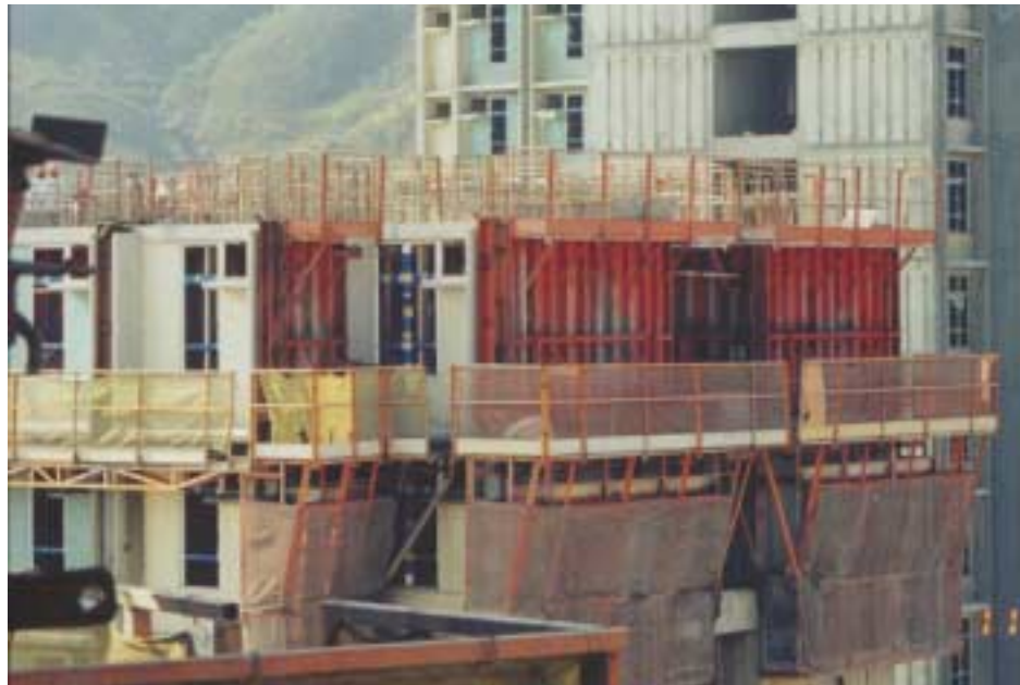
Figure 4.24 Large panel steel formwork
