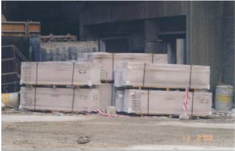
Figure 4.30 Storage of dry wall panels
