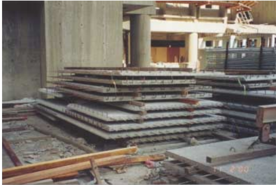
Figure 4.25 Semi-precast slabs
