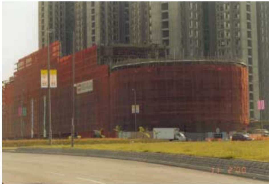
Figure 4.33 Tubular scaffolding for constructing the carport
