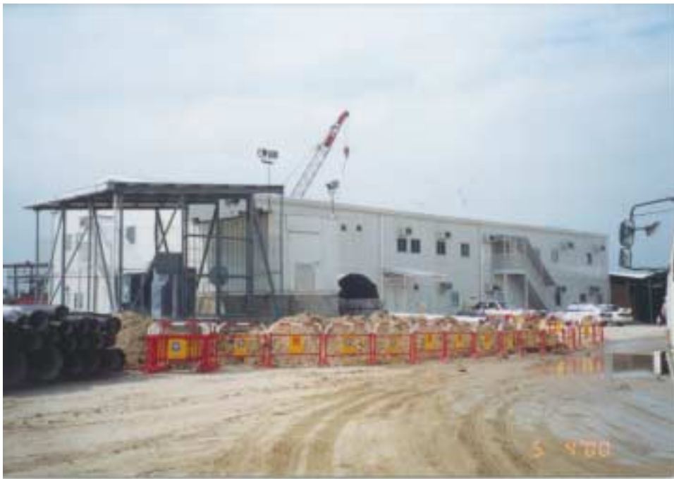
Figure 4.39 Metal panel site office
