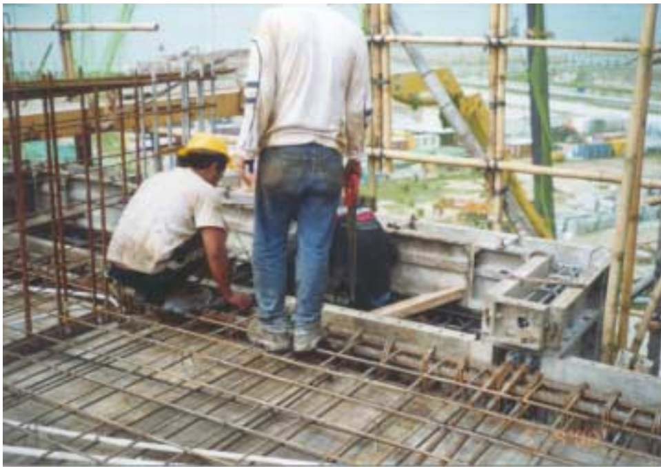
Figure 4.37 Aluminum formwork used to construct the balcony
