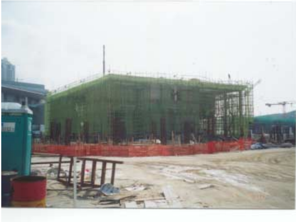
Figure 4.38 Structural steel temporary sales office
