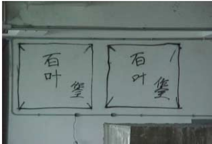
Figure 5.1 Discrepancies in structural and building services drawings led to hacking off of concrete
