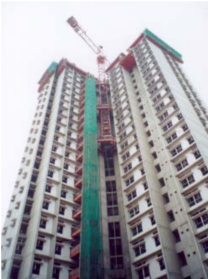
Top: prefabricated facades, general view. Bottom: left, prefabricated facades jointing detail and packaging, right, in situ joint wall.
