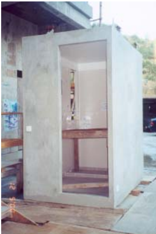
(Left) Prefabricated toilet, (Right) Prefabricated staircases.
