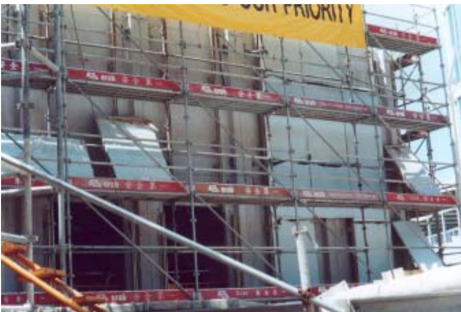
Top and Middle: Metal fromwork. Bottom: Metal scaffolding.
